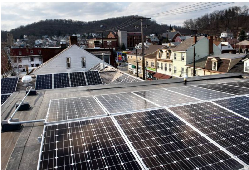
Solar panel installation in Millvale, Pennsylvania
